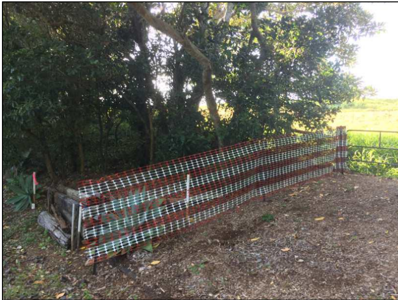
Example of traffic barrier fencing to protect trees.
